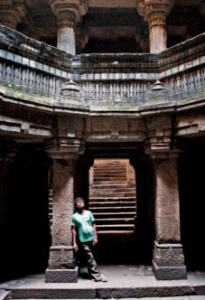
'During our inventory [of wells] many, many locals pleaded for assistance here,' explains Jain, 'so eventually we shifted around ten truck-loads of debris.' The well was slightly deepened to aid its recharging, and the all-masonry construction has benefited from repairs to its walls, columns, eaves, brackets and steps.
